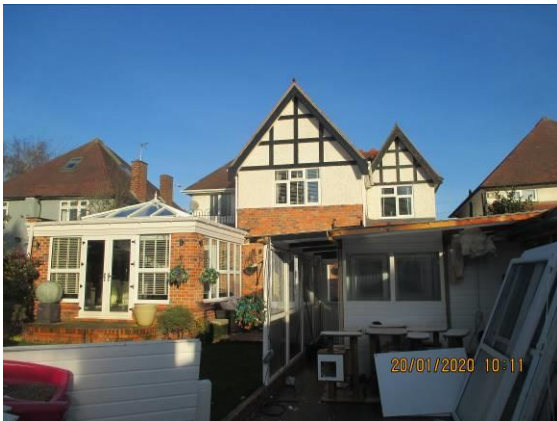
South (rear) elevation (cattery since removed)
